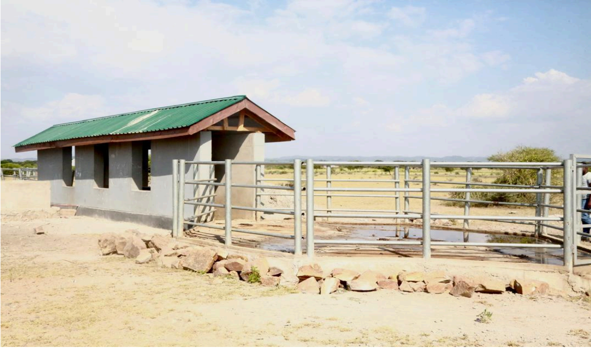
Plate 5.3 Photo showing Dip tanks
