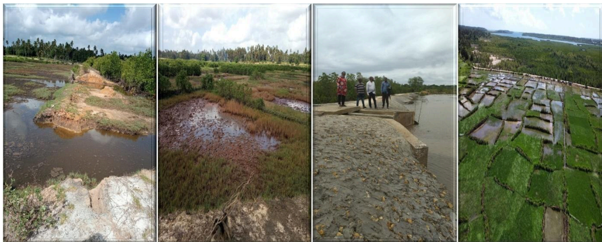
Plate 7.1 Earth Bund technology in Micheweni for controlling sea water intrusion
